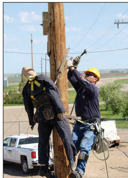
Fairfield lineman John Schwenke demonstrates pole-top rescue.
